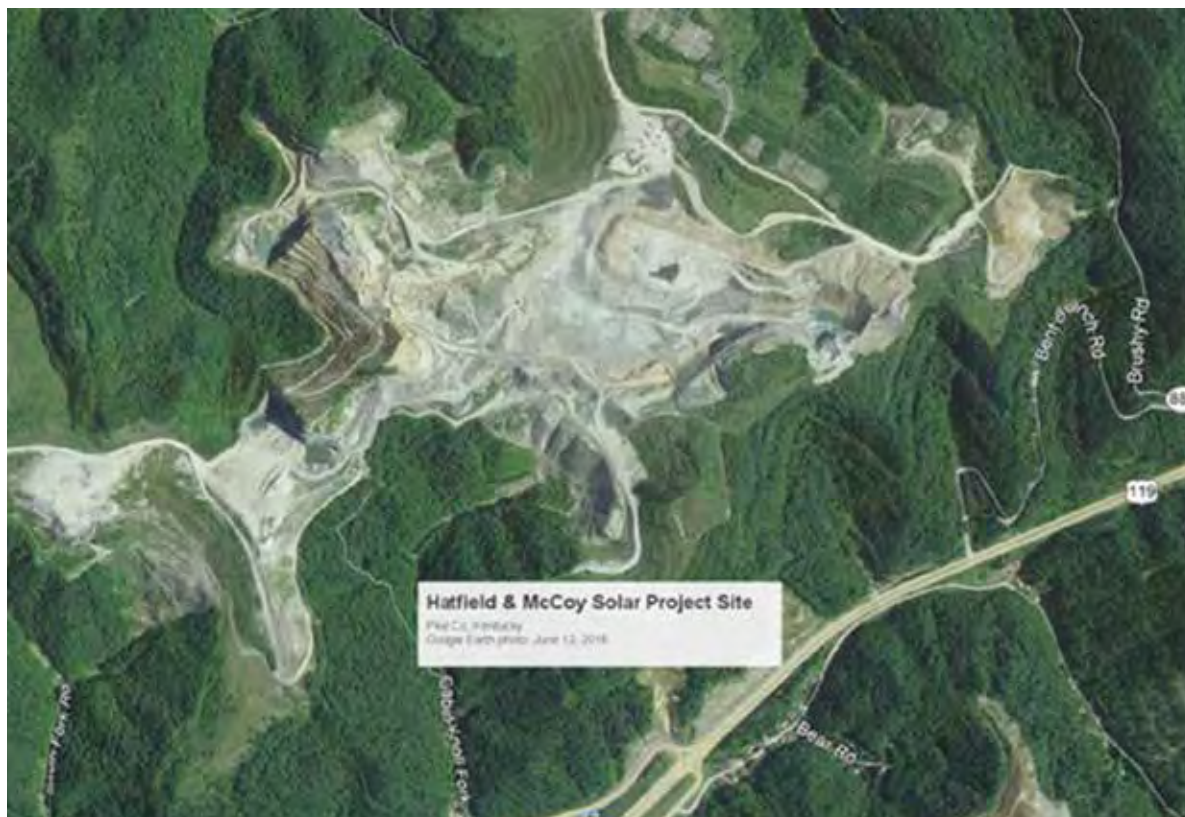
Figure 6 Hatfield & McCoy solar project.
