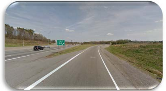
Interstate 40 Looking East Along Exit 138
