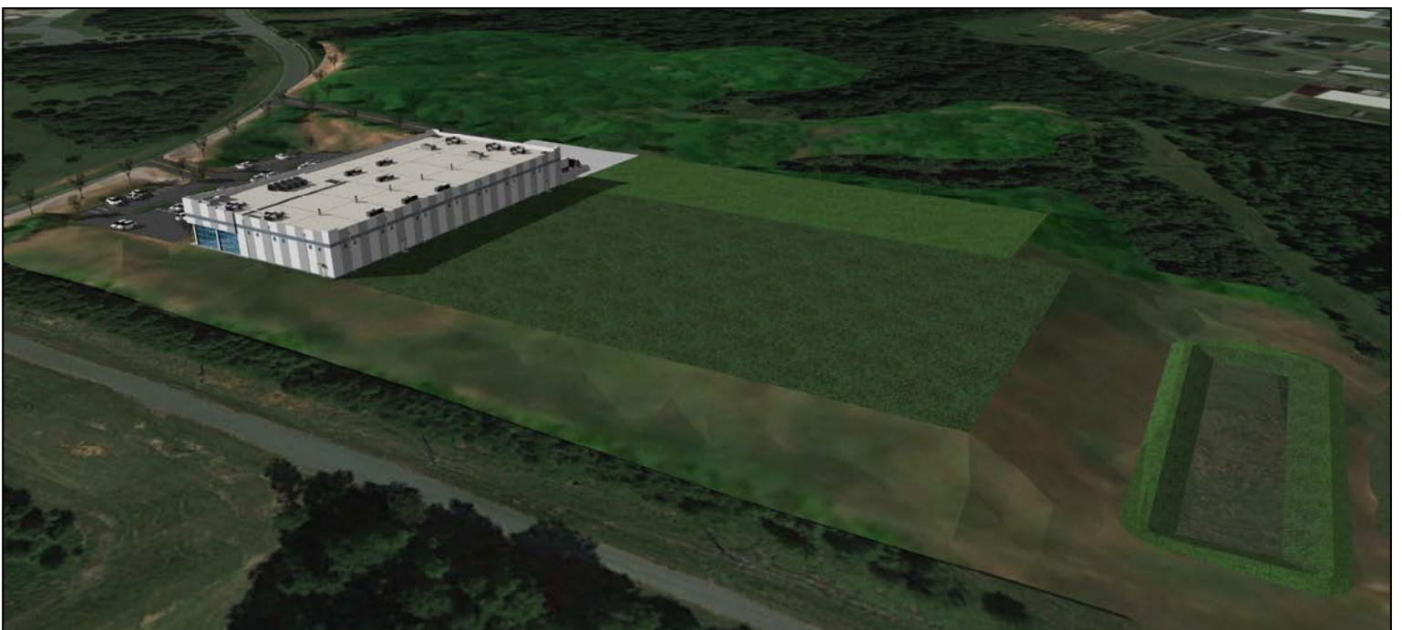
View of Site from the Southeast Looking Northwest from Duke Substation
